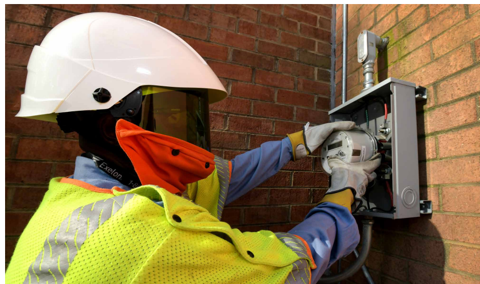
Electric smart meter installation.
